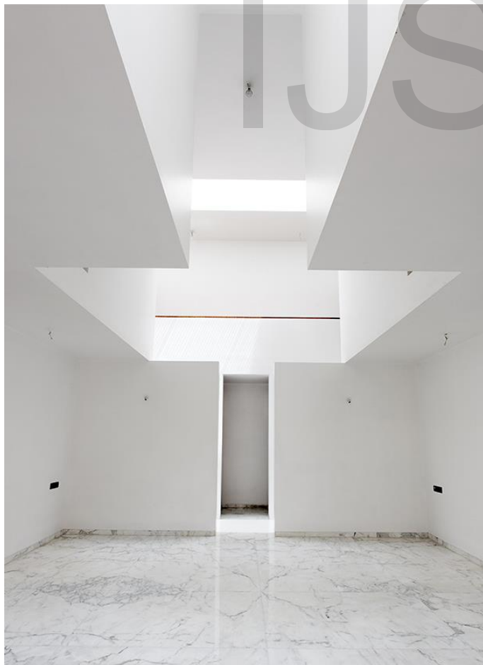
Fig. 4.2.1 Skylight and the double volume volume creating stack ventilation effect Source – Navkar Architects [13]
